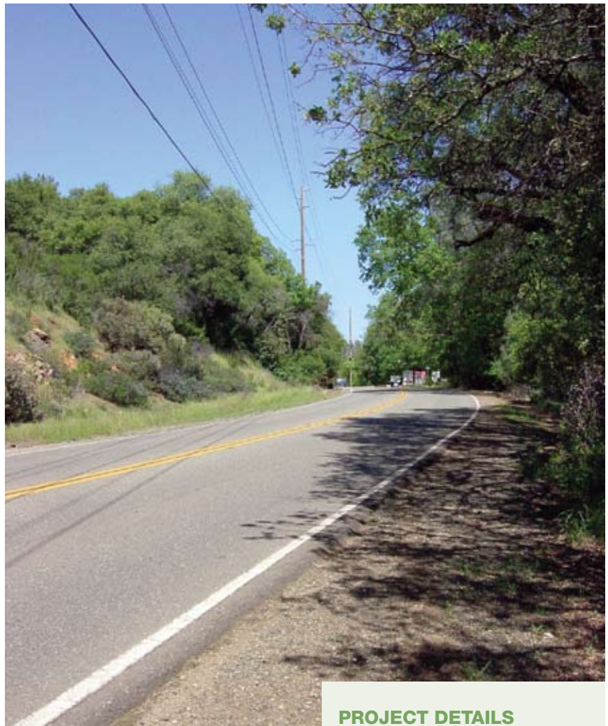
A preconstruction view of EDCDOT's roadway project in Cameron Park, Calif.
